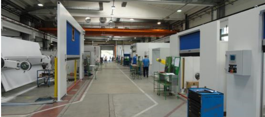
Plant construction and robot systems in Ristro, Slovenia
